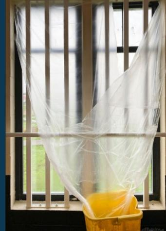
*Left, Deteriorating Building Siding, Right, Temporary Leak Remediation in the MSP Gymnasium Building*
