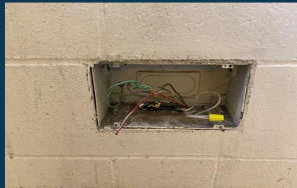
*Left and Right, Former Ground-level Lighting with Exposed Wall Boxes That House Electrical Connections and Wires*
