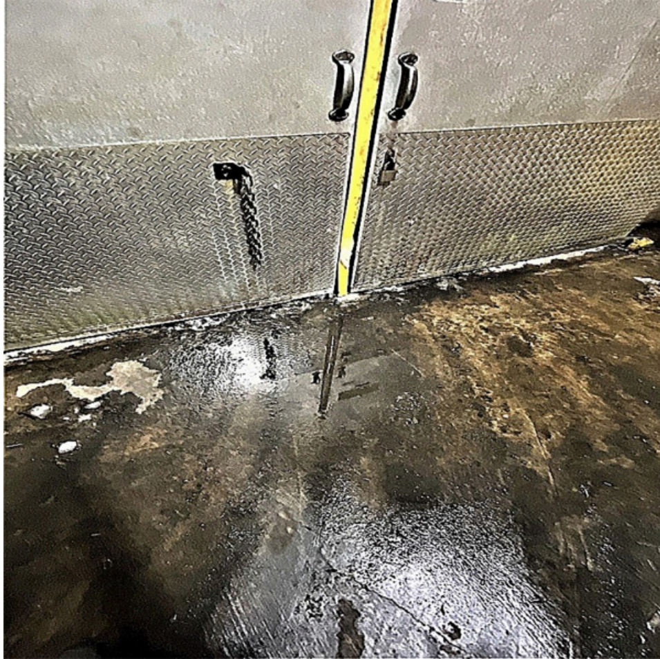
Ice Buildup on the Floor near the Entrance to a Freezer in the Food Storage Warehouse. Source: OIG, June 2024
