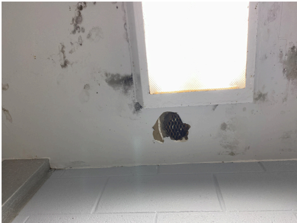
Water Stains and a Hole in the Ceiling of the Camp Kitchen. Source: OIG, June 2024
