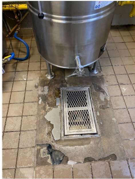
Left and Right, Degraded Floor Tiles near Large Cook Kettles in the Kitchen. Source: OIG, June 2024
