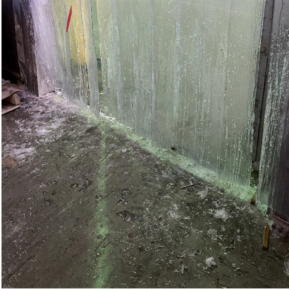
Significant Ice Buildup at the Threshold of the Operational Freezer in the Food Storage Warehouse. Source: OIG, June 2024
