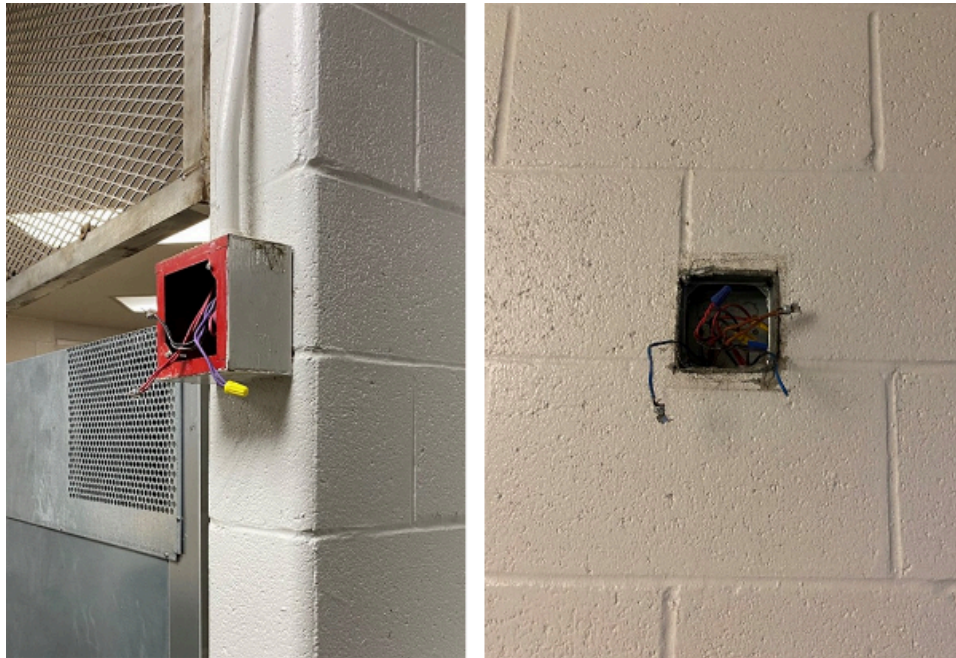
Left, Exposed Electrical Wires Without a Safety Plate in the Secure Cafeteria Serving Area, Right, Exposed Electrical Wires Without a Safety Plate in the Kitchen Area. Source: OIG, June 2024
