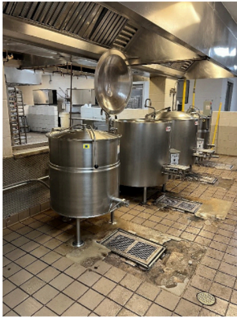
Left and Right, Degraded Floor Tiles near Large Cook Kettles in the Kitchen. Source: OIG, June 2024
